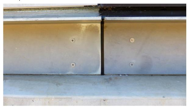
**Figure 1:** A dull grey appearance on some steel beams due to the chemical composition of the steel.
