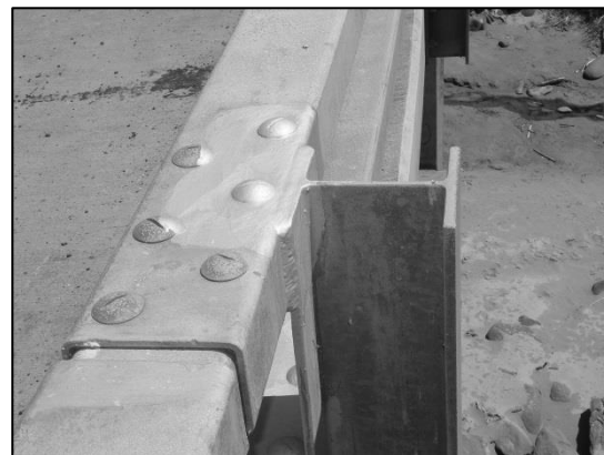
An example of well repaired handrail in a severe corrosive environment (marine).
